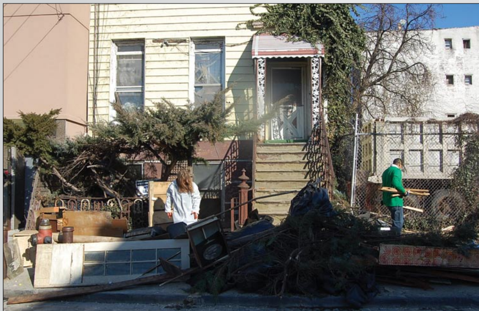
A house in Red Hook, Brooklyn. Basement and first floor were flooded. Three months after the storm it was still uninhabitable.
