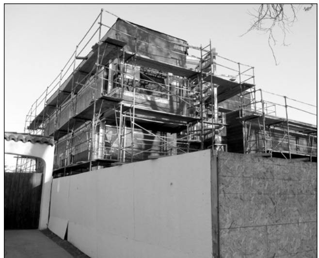
McMansion under construction
