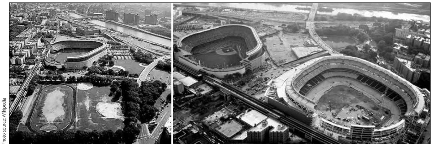
Yankee Stadium site before and during construction of the new facility.
