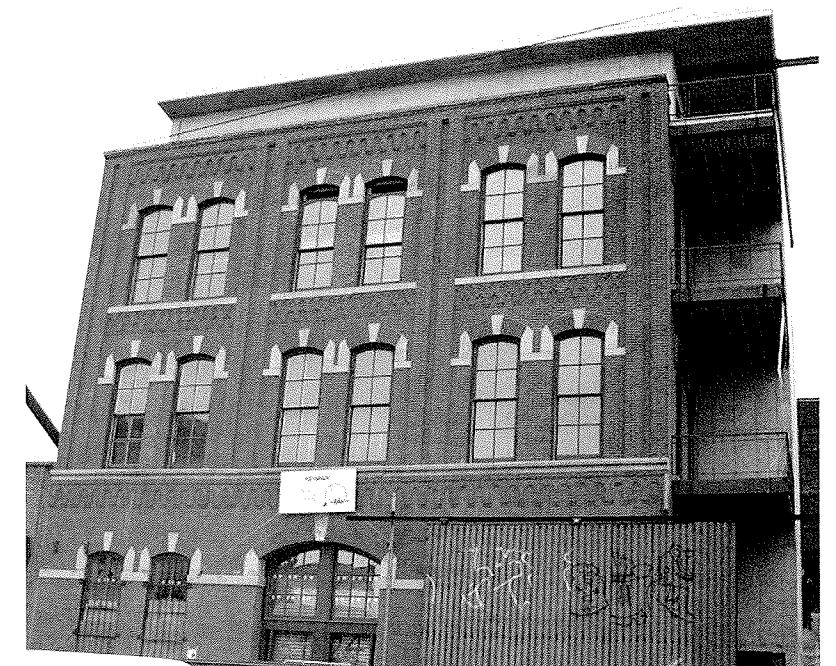
Above: 1024 Dean Street is a 6-unit residential conversion of a previously vacant ice house built in the 1880s in Crown Heights, Brooklyn. Winner of the KeySpan Green Cinderella grant, it incorporates roof-integrated photovoltaics, radiant in-floor heating, 2300 square feet of green roof and extensive use of reclaimed wood.
